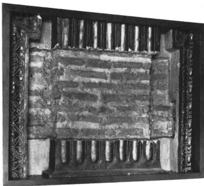
Fig. 41. S. Maria Maggiore, Pilaster of clerestorey denuded of sixteenth century revetment (from plaster cast)
